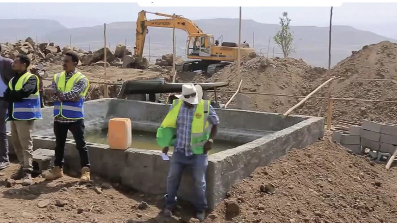
Workers at the new building site
